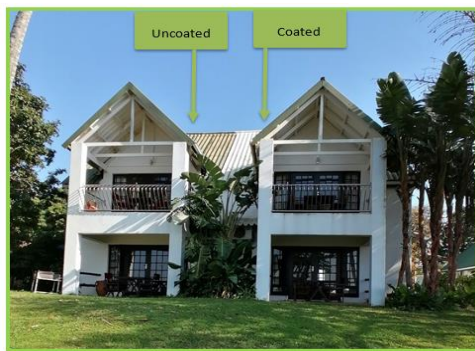
Figure 2: View of adjoining application and reference bungalow
