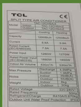
Figure 6: Nameplate of HVAC units installed in experiment bungalows
